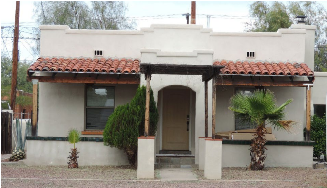
Covered entryway and extended porch with wood posts
