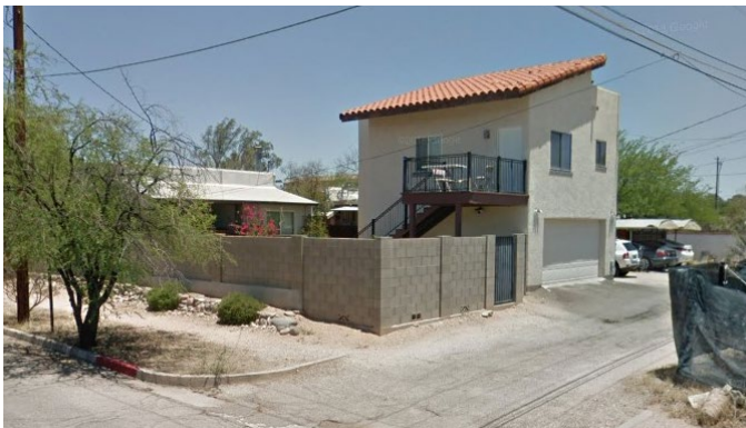
Vehicle access and storage via back alley
