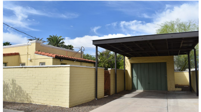
Carport behind house
