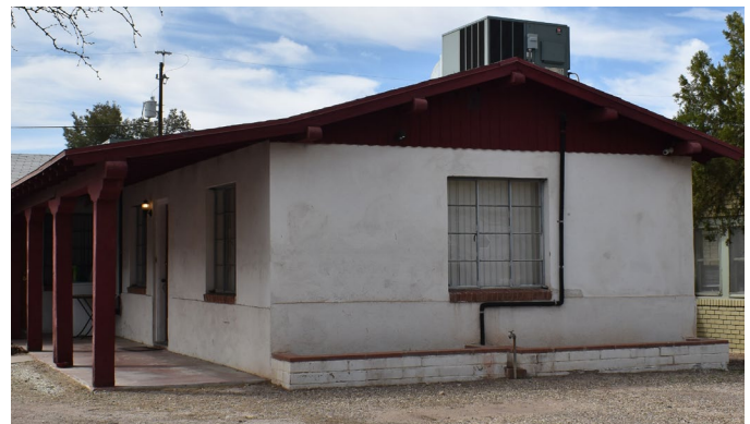
Multi-light steel casement window
