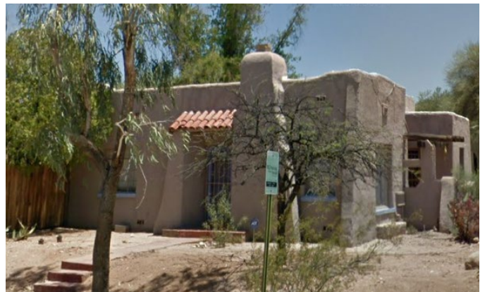
Flat roof with rounded parapet and asphalt
