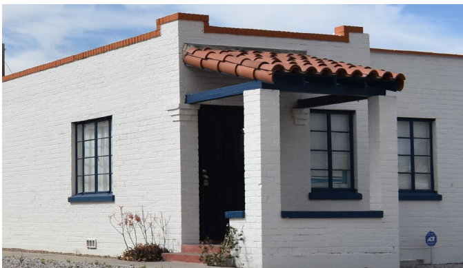
Multi-light steel casement windows
