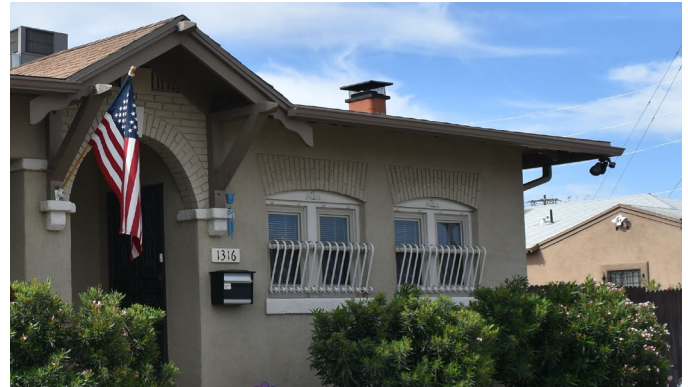
Grouped double-hung sash windows with decorative wrought iron bar guards
