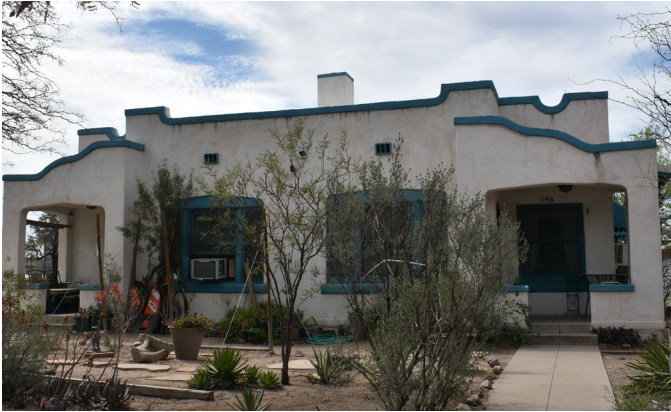
Flat roof with stepped parapet and asphalt
