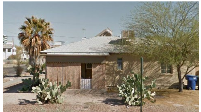
Enclosure has altered the character-defining porch and risks a loss of integrity.
