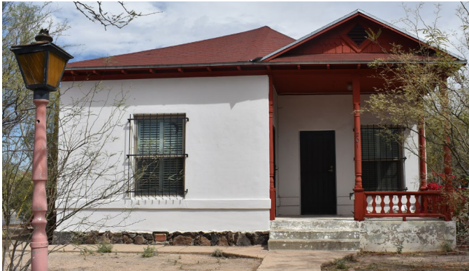
Double-hung sash window with bar guard
